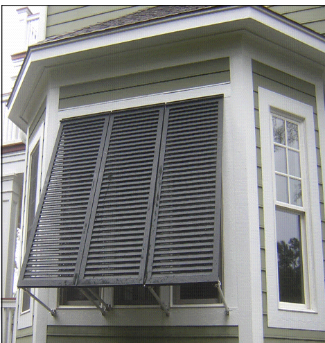
This triple window has three separate bahamas, each with a pair of stand-out arms. Note that the center bahamas' arms are attached higher than the two outsides sets. This is to allow inserting and removing the locking pins.
