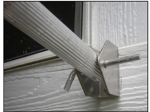
The locking pins and standout bars are removed when the shutter is going to be closed.
