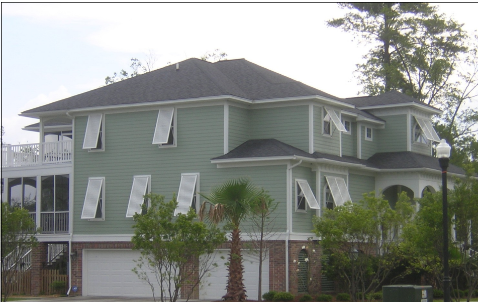
Impact-rated bahamas offer several benefits. They provide shade, can be closed from inside the house and they add a tropical touch of a house.
